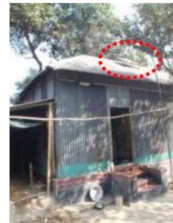
SHS Installed House
